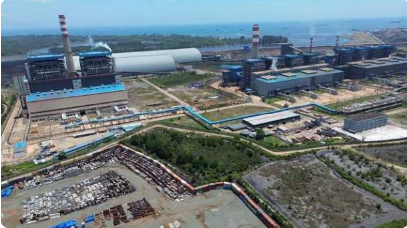
The Captive Coal-Fired Power Plant (PLTU) of PT Obsidian Stainless Steel (OSS), located in Tani Indah Village, Kapoiala District, Konawe Regency, Southeast Sulawesi. (Photo: Courtesy)
